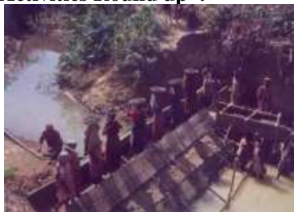
Construction of Check Dams
